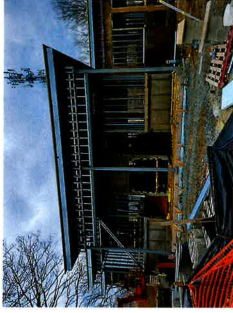
Elevator Blocking and Exterior Framing
