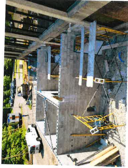
Masonry Walls for Rear Addition – 1 st Floor Complete
